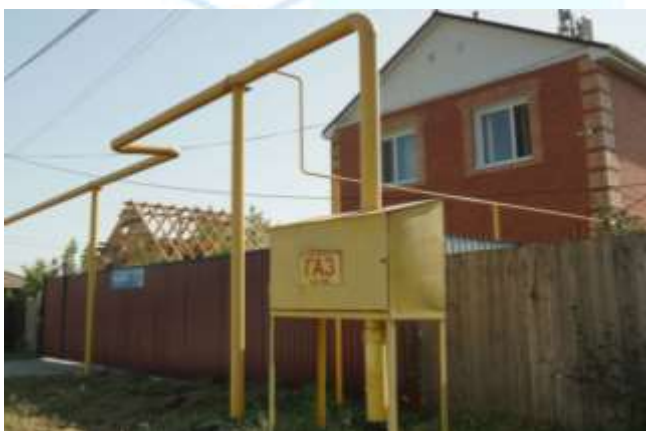
2 – picture. Installation of gas pipelines in residential buildings
