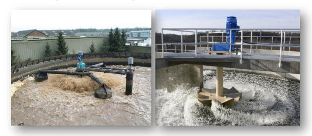
Mechanical aerators have a number of advantages over pneumatic ones since their installation does not require the construction and operation of blower stations, and air supply communications, they are easy to manufacture and operate and have a high oxidizing ability. Their disadvantages include the need for a large number of aerators to be installed with large structures, the need for scarce equipment (gearboxes, gear motors), as well as insufficiently high reliability of operation.
